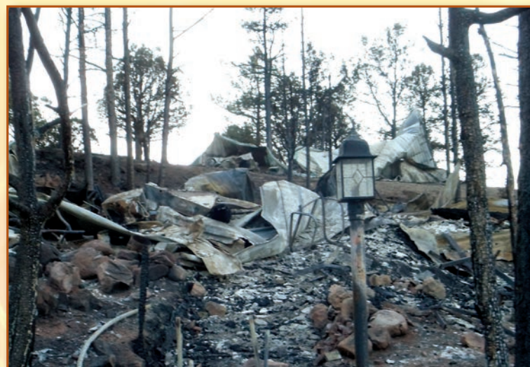
The Little Bear Fire destroyed this home and more than 250 other structures when it burned near Ruidoso in 2012. Photo courtesy of Kelly J. Hamilton, Southwest Border Food Protection and Emergency Preparedness Center.
